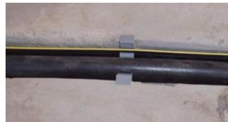
数据通讯系统集成在初级电缆中 Data communication system integrated in primary cable
